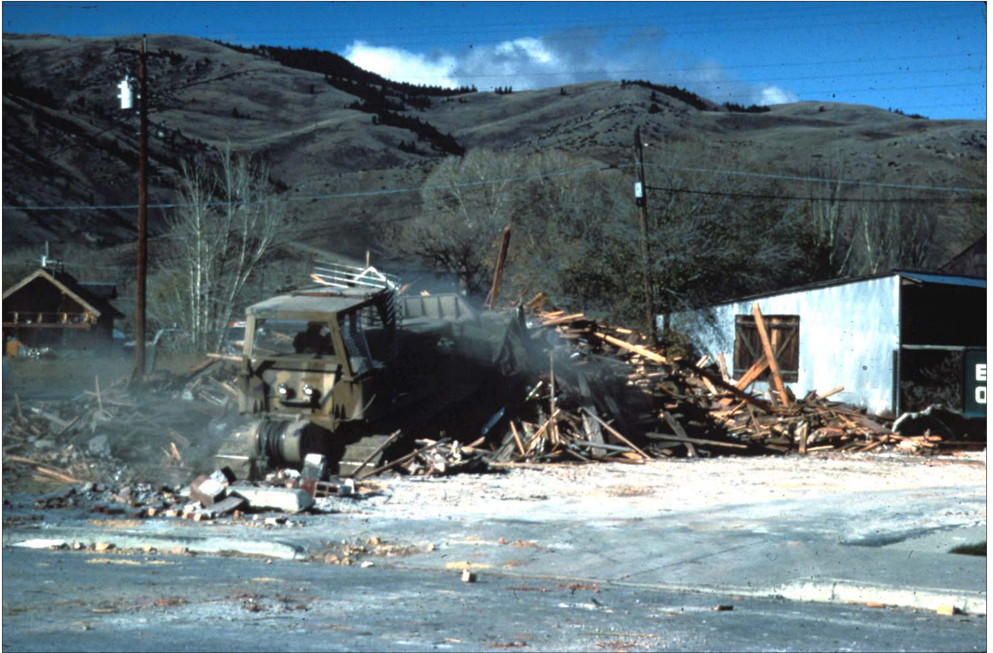
Destroyed buildings in Mackay, damaged by quake.
